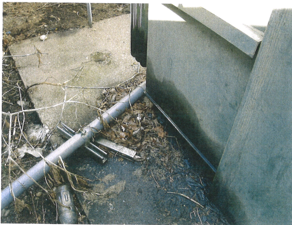
Photo 10 – Staining was observed in the vicinity of the electrical transformer south of the clubhouse.
