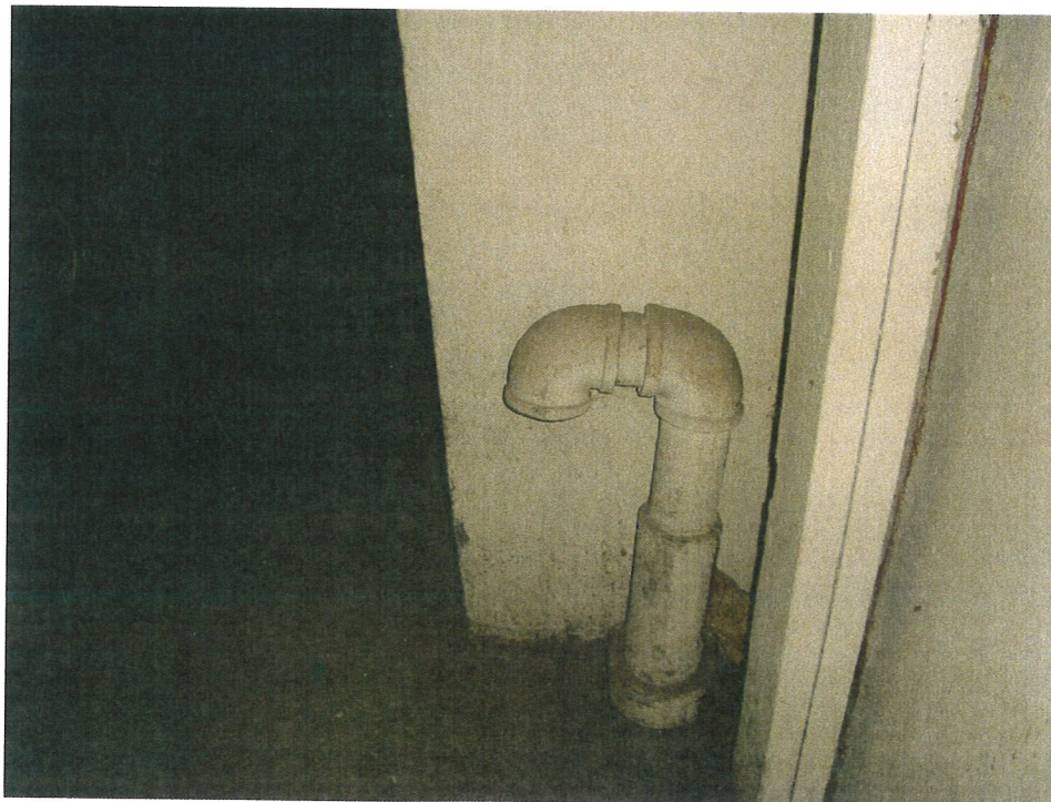
Photo 12 – View of the sewer vent which was observed in the Pro-Shop.
